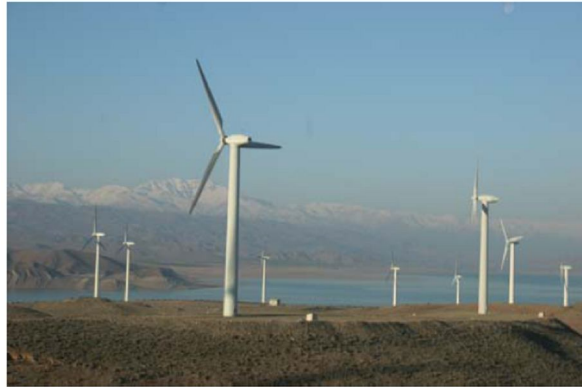
Figure 1: The Manjil wind farm
